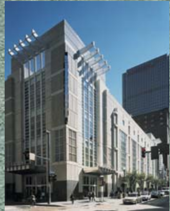
Lazarus Department Store, Use of precast cladding allowed architects to model the façade
